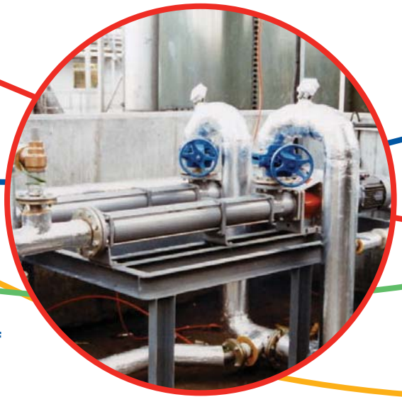
Pumping of slurry mix
